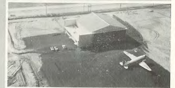
Initial unit of flight test facility
